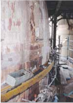
2. Bottom rail with top rail mounting brackets in position
