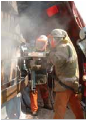
10. Cutting the refractory
