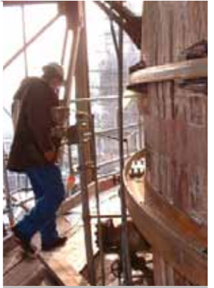
5. Top and bottom rails ready for dressing
