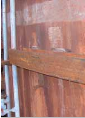
1. Bottom rail showing secure welds
